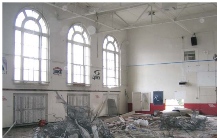
January 2006: The original gymnasium in the 1926 building begins its facelift.
