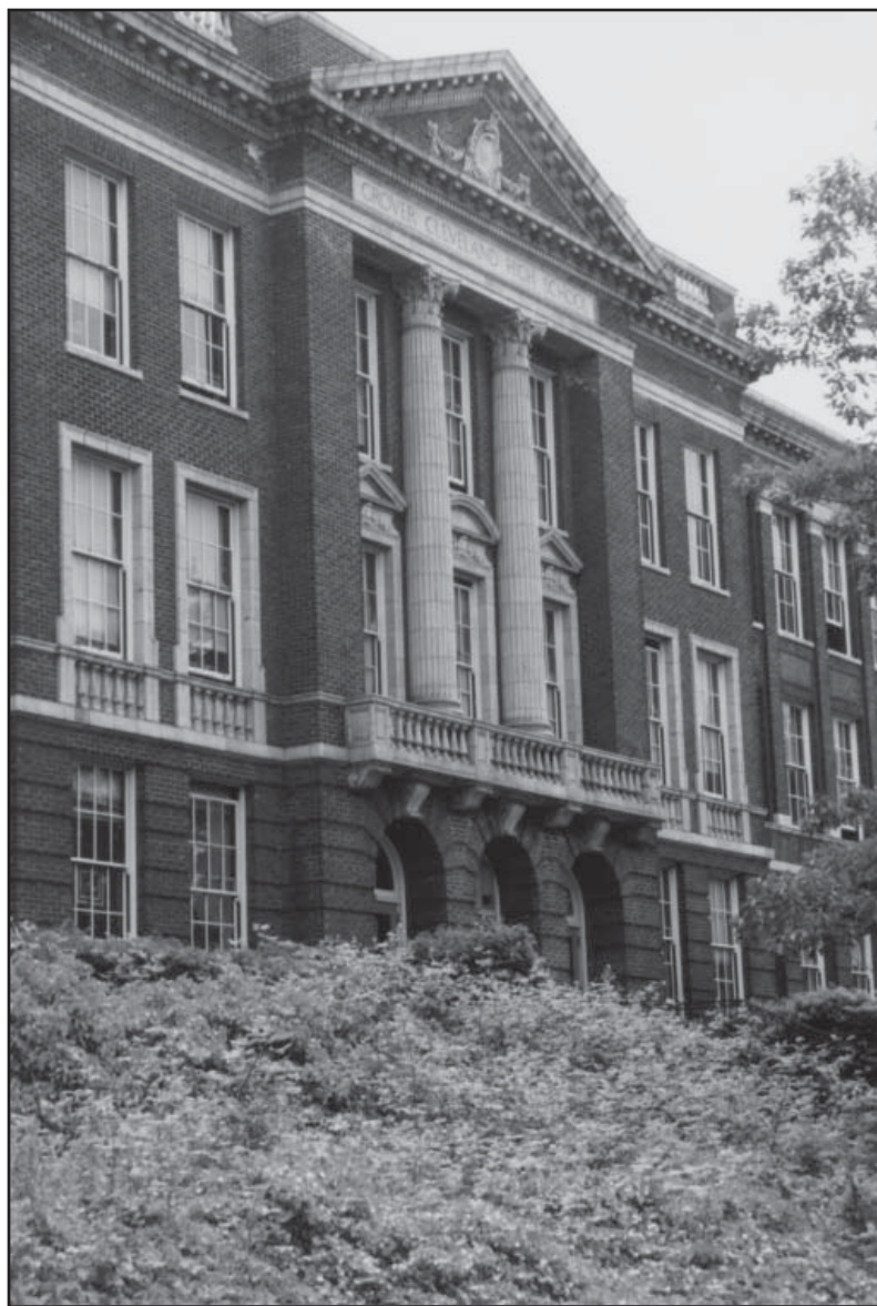
The original Cleveland High School facade
