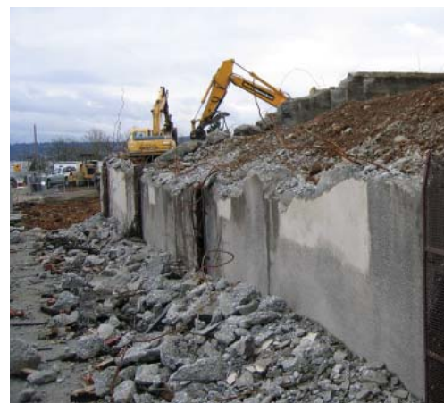
January 2006: The two-story wall on 15th Avenue South is removed.
