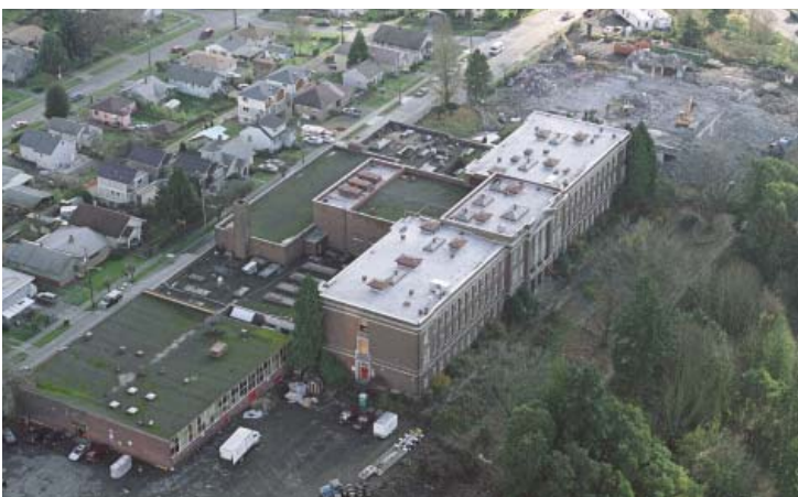
November 2005: Aerial photo showing the removal of the 1969 gymnasium building.
