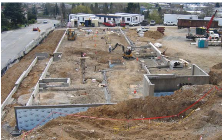
March 2006: The new academic building's foundation is poured.
